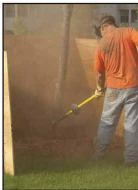
Airspade tool used to blow soil away
